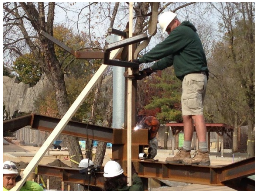
Welding the last piece onto the frame
